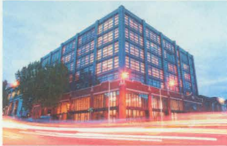
Sunset Electric is located at 1111 E. Pine St. It is one of the few LEED-Platinum apartment communities in the Pacific Northwest.
